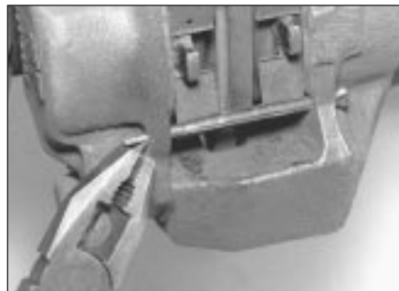
7.10 Spread the ends of the split pins to retain them in position
